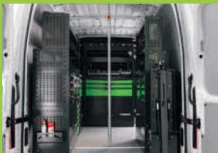
POLES STOP LOAD
